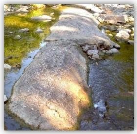
Exposed sanitary sewer crossing upstream of Dry Creek WWTP
