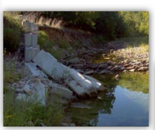
Concrete blocks installed in an attempt to stabilize the stream bank near Duke Energy gas main
